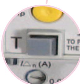
Test Button (to test the residual current detection and tripping system)
